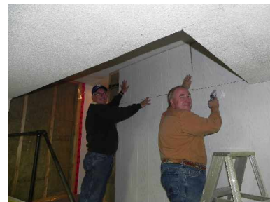
Gord Fraser and Ron Towns put up vapour barrier John Hodder and Roy Eaton install panelling The brethren got together and made quick work to the banquet room renovations that included new walls, panelling and a ventilation system.
