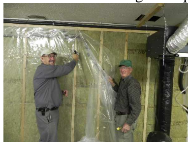
Gord Fraser and Ron Towns put up vapour barrier John Hodder and Roy Eaton install panelling The brethren got together and made quick work to the banquet room renovations that included new walls, panelling and a ventilation system.
